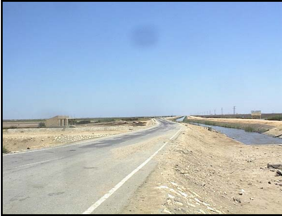
Photo 11 “proposed crossing of the canal branch no7 from El-Sheikh Gaber canal and the parallel small road
