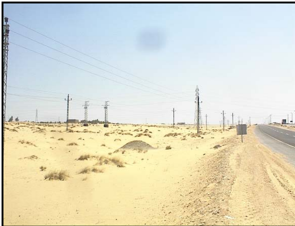
Photos 15, 16 “El-Qantara – El-Areish road parallel to the proposed pipeline from the north direction behind Romana village on the road”
