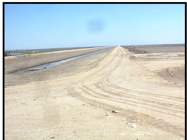
Photo 8, 9, &10 “proposed crossing of the canal branch no1, 3, and 5 from El-Sheikh Gaber canal and the parallel small roads”
