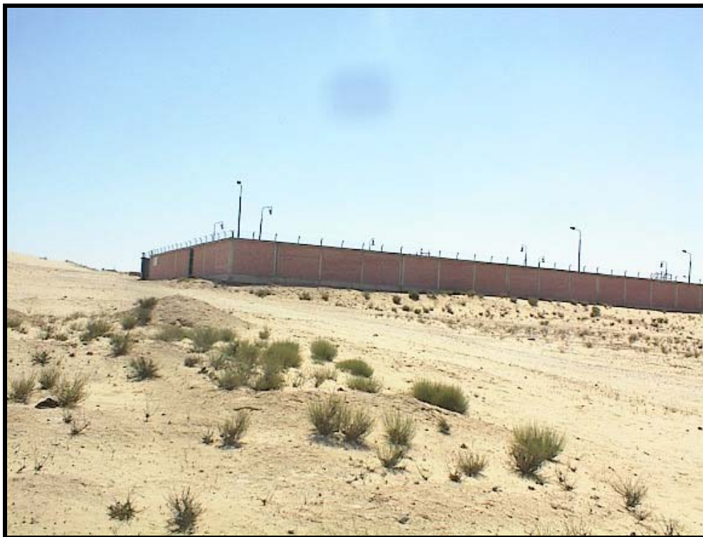
Photos 29, & 30 “End point of Loop 2 of the proposed Abr Sinai pipeline”
