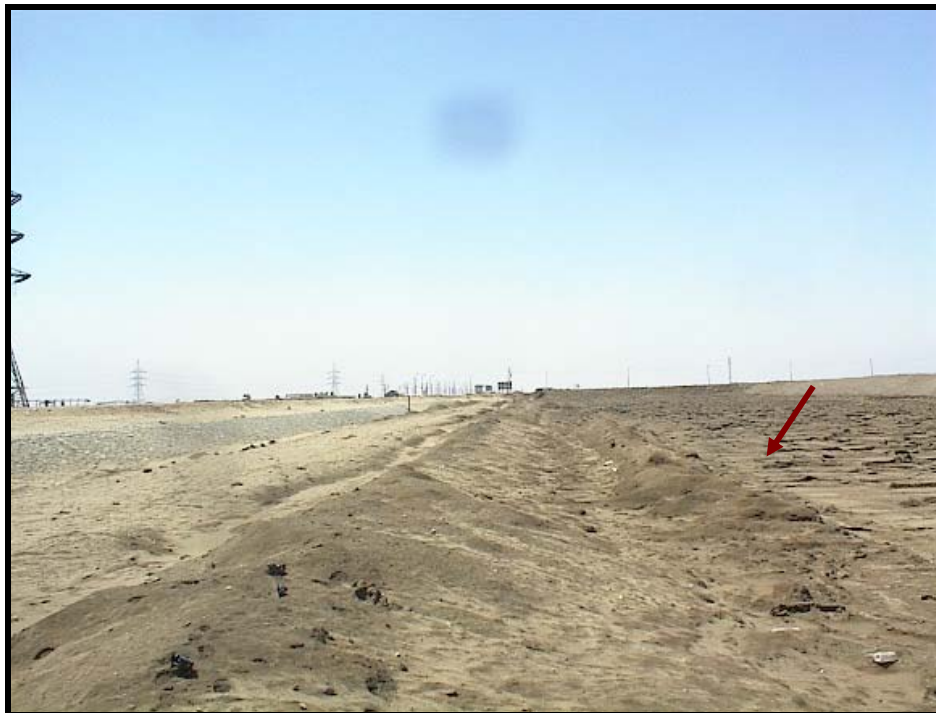
Photo 2 “The proposed pipeline route for 400 m parallel to the existed pipeline El-Tena East- Ouen Mousa”
