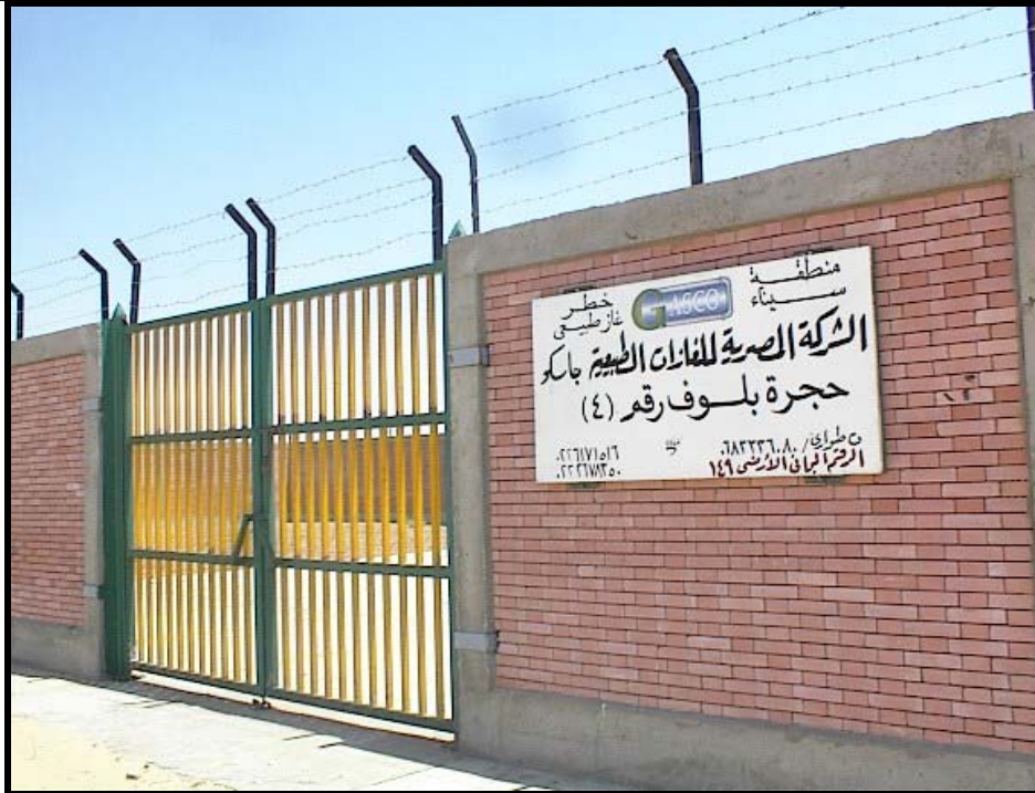
Photo 19 “Start point of Loop 2 of the proposed pipeline, showing valve room No 4 at Bair El-Abd along the existed pipeline route”
