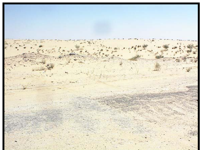
Photos 21, 22, &23 “proposed pipeline route parallel to the existed pipeline in the desert area 3 km South El-Qantara – El-Areish road”
