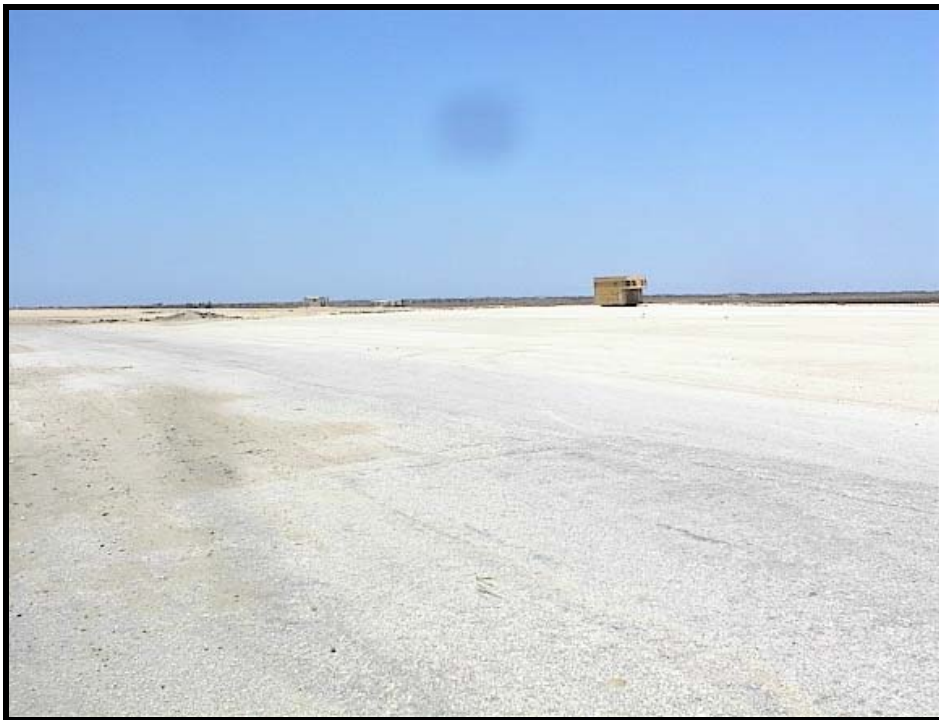
Photos 13, & 14 “proposed pipeline crossing of the old temporary airstrip. parallel to El-Sheikh Gaber Canal”
