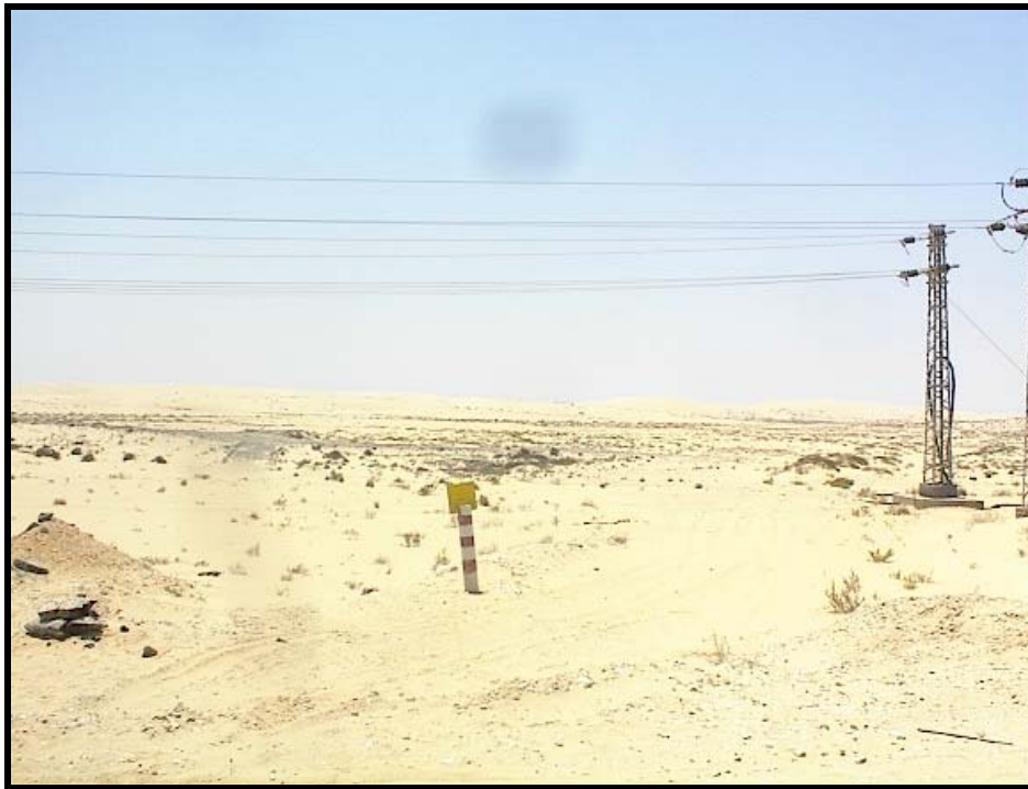
Photo 17 “the proposed pipeline parallel to the existed Abr Sinai old pipeline”
