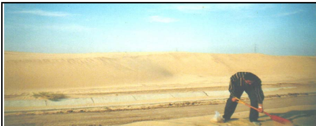
4.7 Small canal of irrigation from the El-Salam canal partially covered by active sand dunes.
