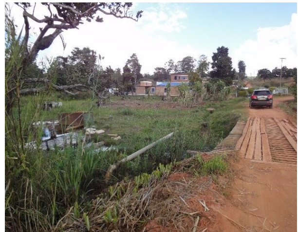
Figure 2 – Road bridge, WTP, and weir u/s on the left
