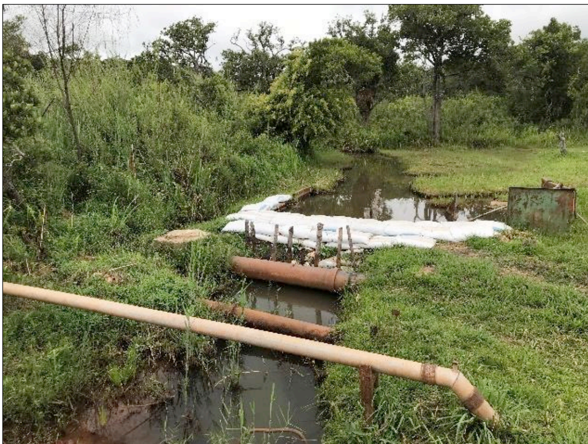
Figure 1.1: Existing makeshift kind of weir near the Mzuzu WTP
