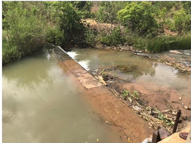
Figure 2 – Existing weir, viewed from the right bank
