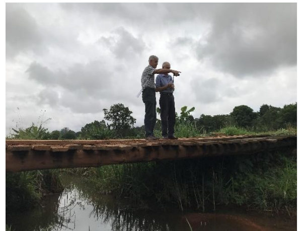
Figure 5 Road bridge, viewed from u/s
