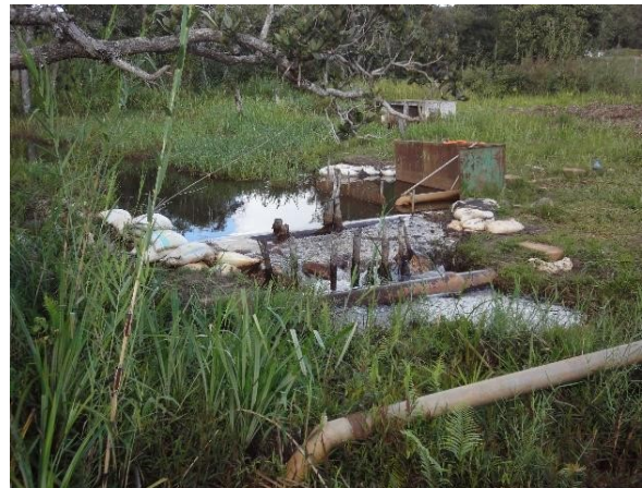
Figure 4 – Existing weir viewed from d/s RB
