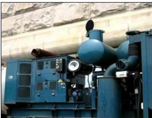
Figure 7.2.4.1.1: Muffler system
