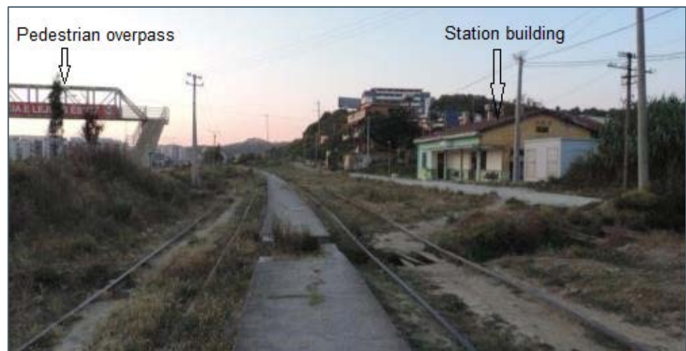
Figure 3-8_Pedestrian overpass that serves only the motorway – Golem station
