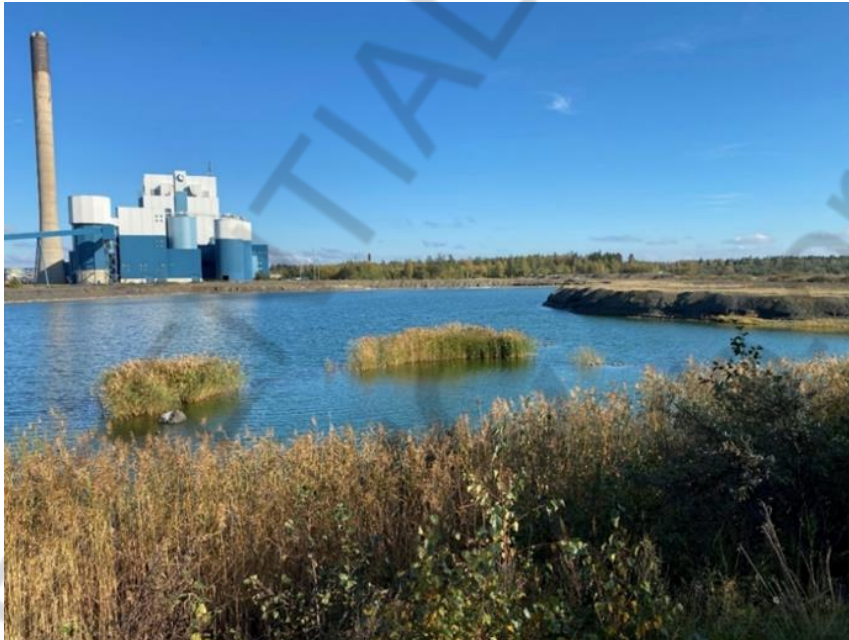
Figure 6.2-2. Water pond and filling area on the eastern edge of the VRP area. The Meri-Pori power station can be seen in the background. Photo taken towards northeast. Point B in Figure 6.2-4.
