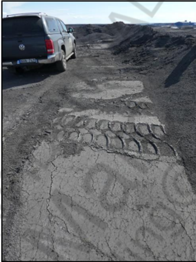
Figure 6.5-5. Compact surface of a slag stockpile in Luleå.
