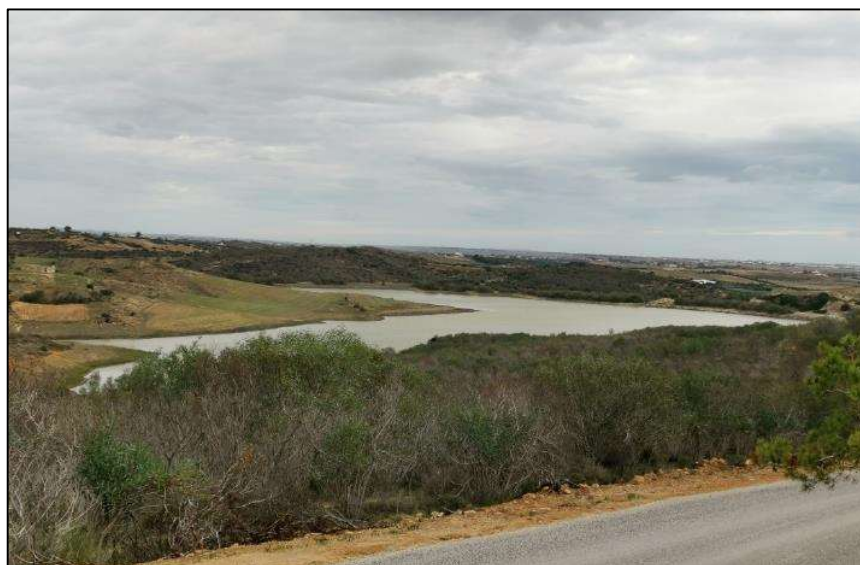
Figure 37 : The Chiba Dam (36°41'41.99"N, 10°45'48.78"E)
