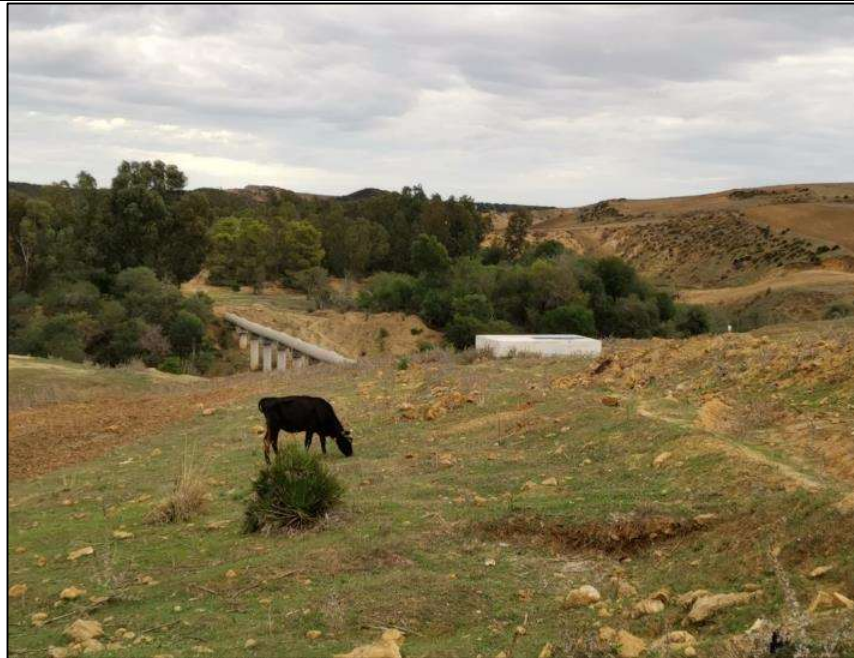
Figure 38 : Water pipeline near the Chiba dam
