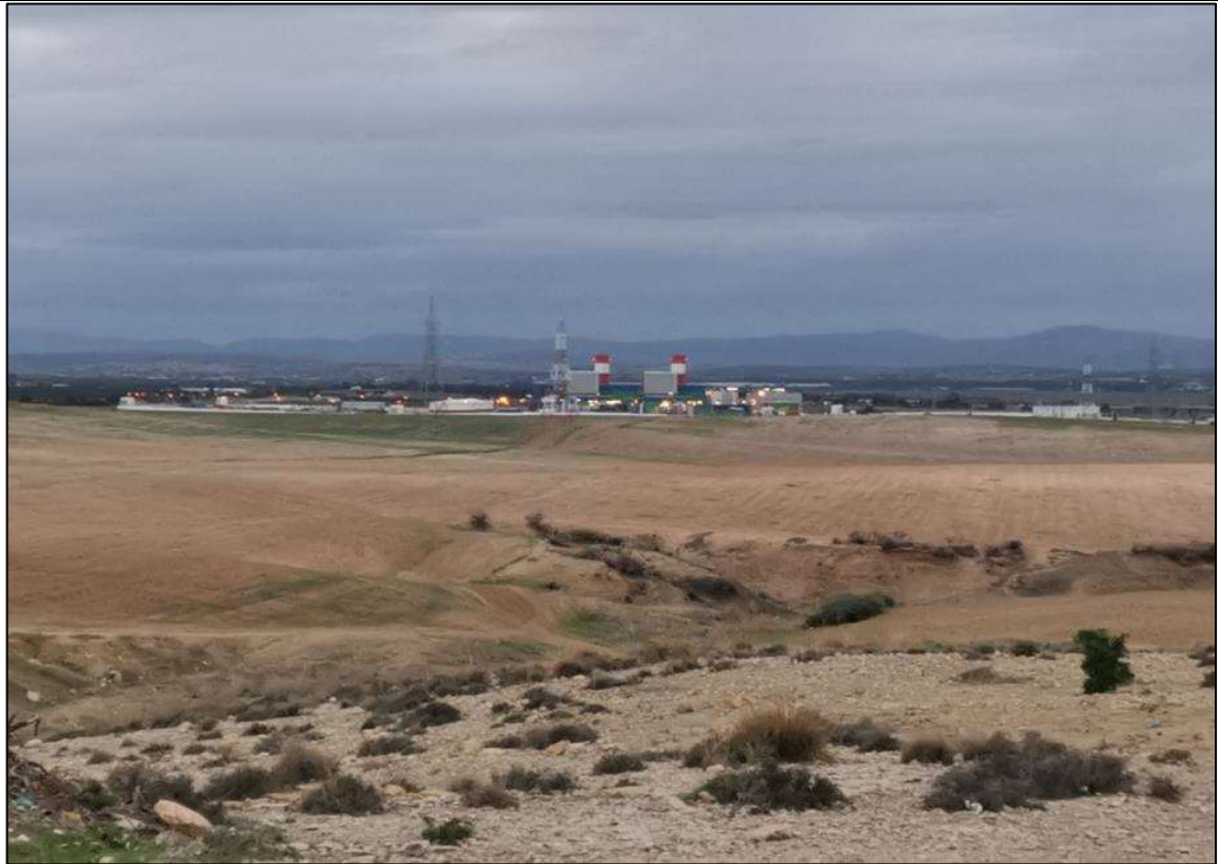
Figure 65 : The Mornaguia station (36°40'41.57"N, 9°55'25.05"E)
