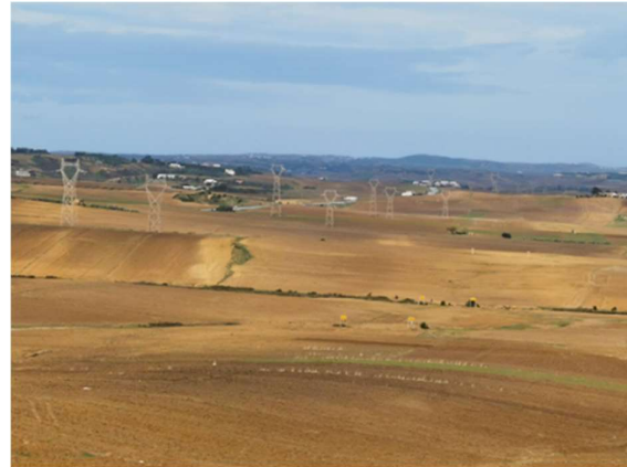
Two existing power transmission lines installed on agricultural land between El Mida et Menzel Temime
