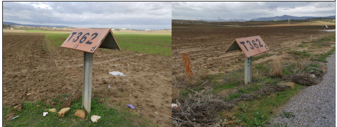
Figure 33 : Markers for the gas pipeline Algeria- Italy (SERGAZ Company)
