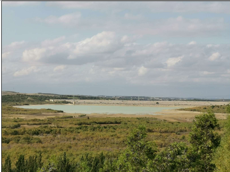
Figure 57 : The ELHAMMA Dam (36°35'3.15"N, 10°18'11.20"E)
