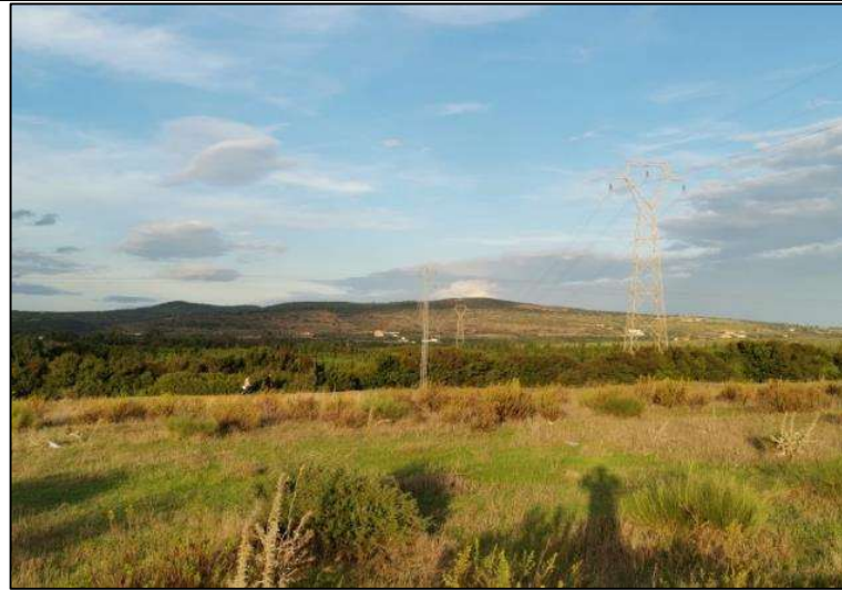
Figure 43 : S10-S11 section: first plan open land with natural vegetation and second plan we can see the citrus plantations and presence of the 90 kV OHL line of Menzel Temime and Grombalia
