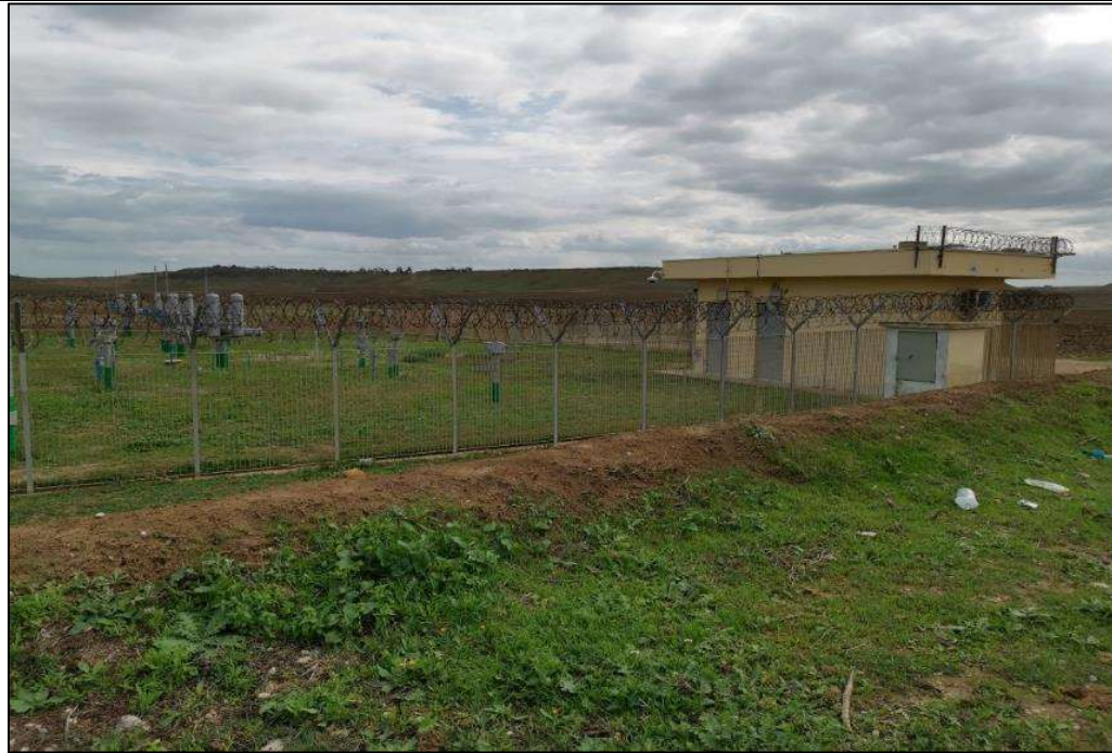
Figure 34 : The Gas station observed (36°45'17.83"N, 10°51'1.92"E)
