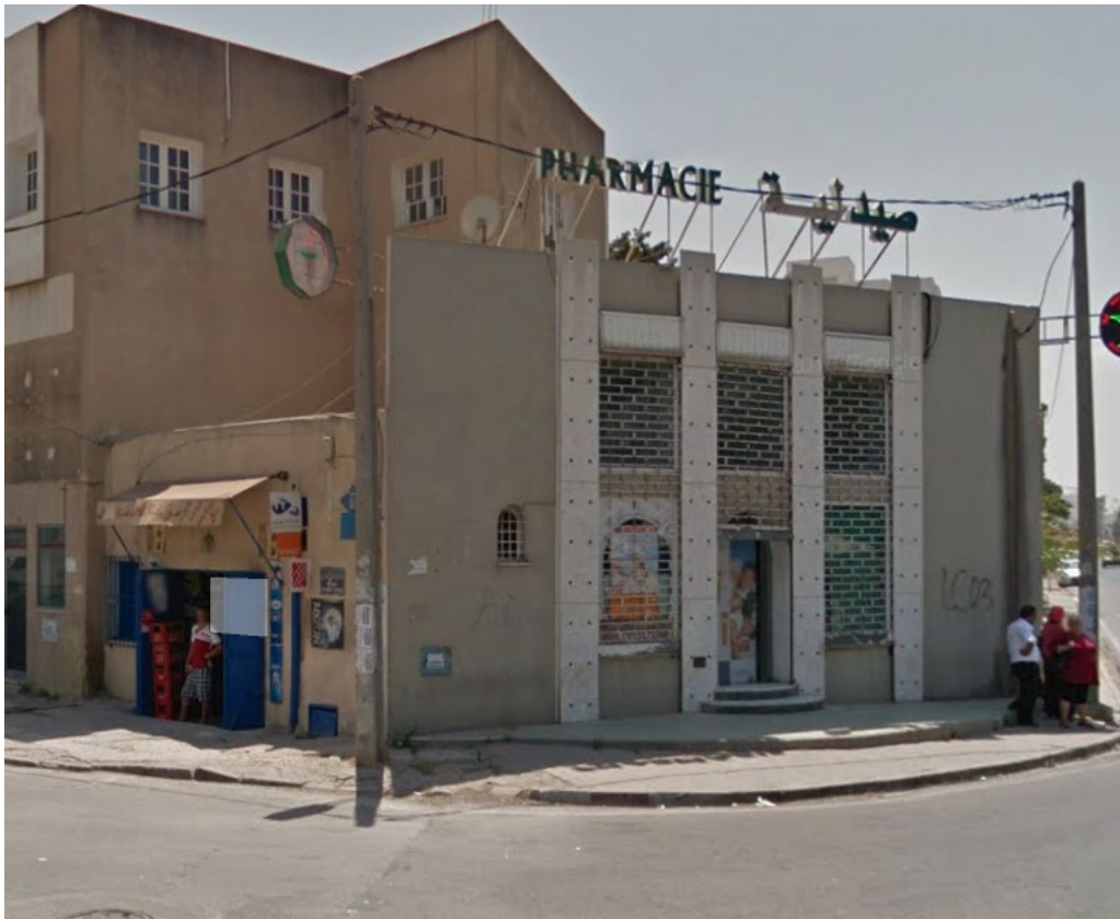
Photo of the store and pharmacy to be demolished
