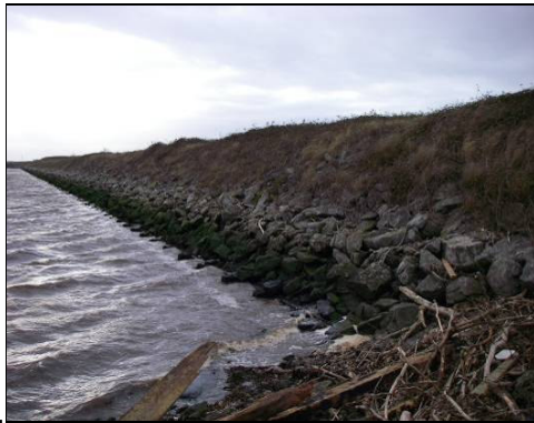
Photo 4.1: Boulder defences of the River Tees North Bank
