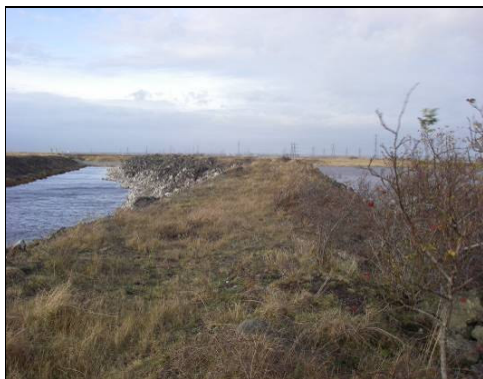
Photo 4.3: Boulder embankments in the SE corner of the Reclamation Pond
