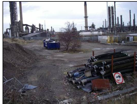
Photo 4.8: Lay down areas and portacabin offices within the Sabic Refinery Site
