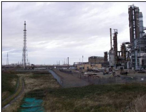
Photo 4.7: Hard standing lay down areas within the Sabic Refinery Site
