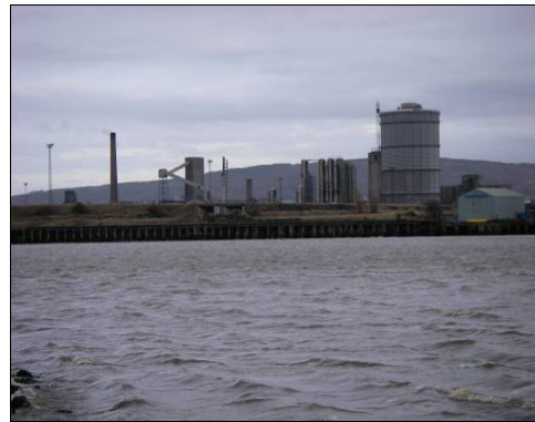
Photo 4.2: Wharf frontage along the River Tees South Bank
