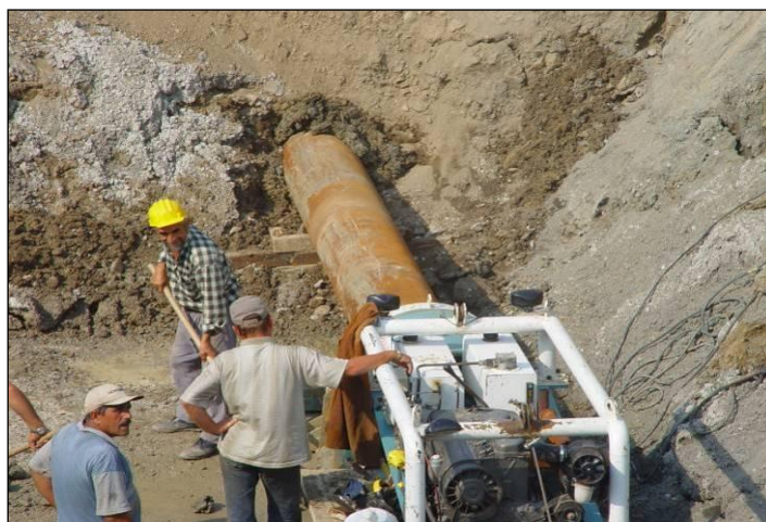
Photo II.4 The Work in which Thrust Boring Method Was Used
