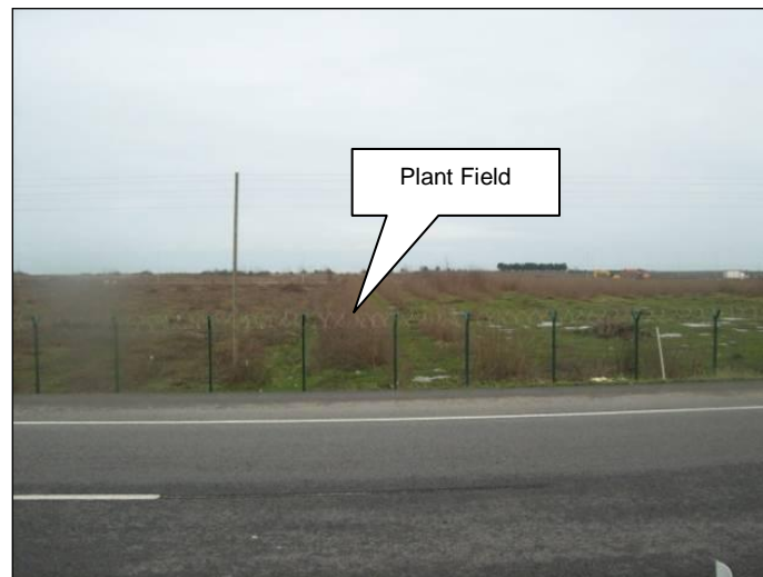
Photo II.2 Natural Gas Pipeline Ending Point
