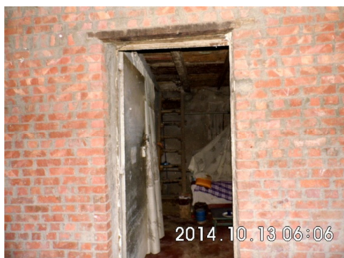
Photo 2-3: Upgrading of walls
