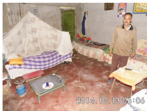
Photo 2-4: Upgrading of floors
